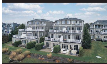
40 Trott Blvd, Unit 205, Collingwood
